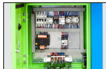
Control panel box.
