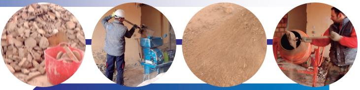
The debris processed by the TRITON is transformed in sand, that can be reused to produce mortar/concrete.
