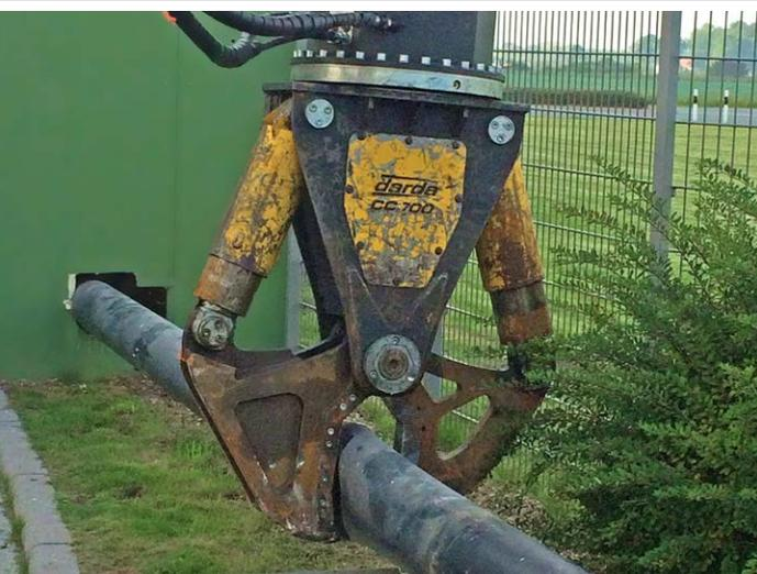
Risk of explosion in an underground cavern storage facility – how can the aboveground pipe system be safely and quickly dismantled? The Darda CC700 S Steel Shear makes this type of work possible.
