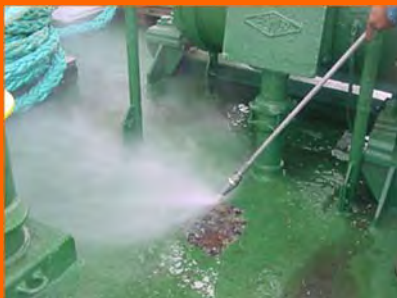
Blasting- Rotating Nozzle
