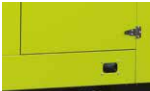
Opening for fuel pipes
