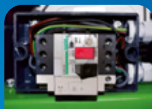
Magneto-thermic ON/OFF switch
