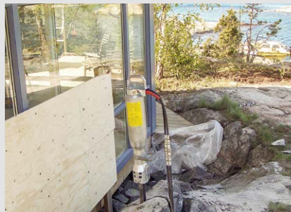
Demolition of rock and natural stone
