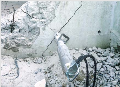
Demolition of concrete and reinforced concrete
