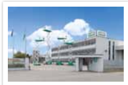
IMER Access (Aerial Platforms) Pegognaga (Mantua), Italy
