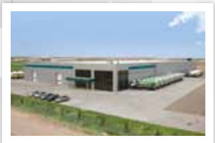
Concrete Machinery (Truck Mixers) Aksaray, Turkey
