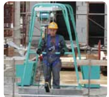
Gantry for stand hoists
